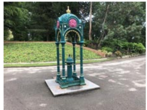
William Hall Water Fountain
