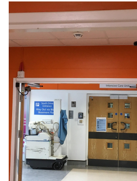
3. Photo Intensive Care Unit near the lift
